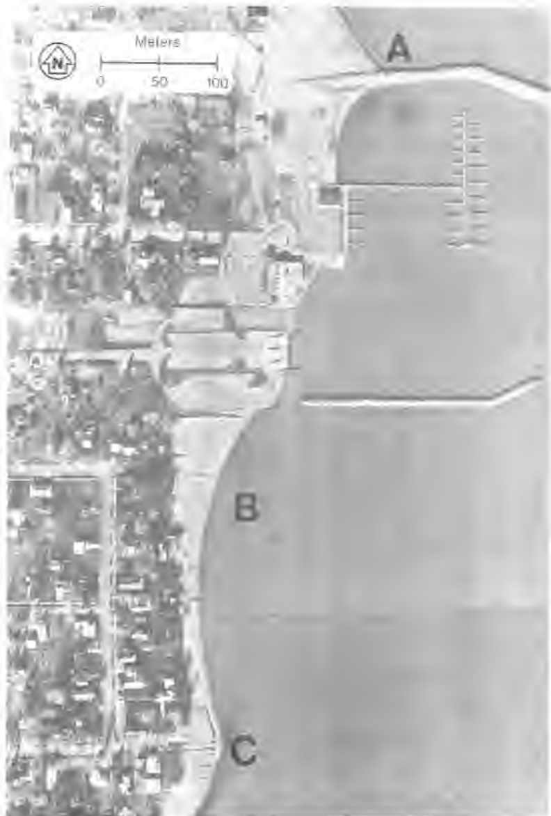
Figure 5. Lexington Harbor, 6 December 1981. A is the accretion area 14 months after removal of about 19,000 cubic meters of beach sediment; B is the part of the feeder beach that received the 19,000 cubic meters of beach sediment from the accretion area; C is the part of the feeder beach 14 months after receiving about 35,000 cubic meters of sediment from a nearby land borrow site.
